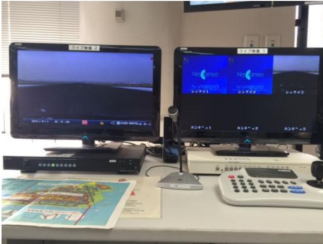
Monitoring of the airport in the control room
