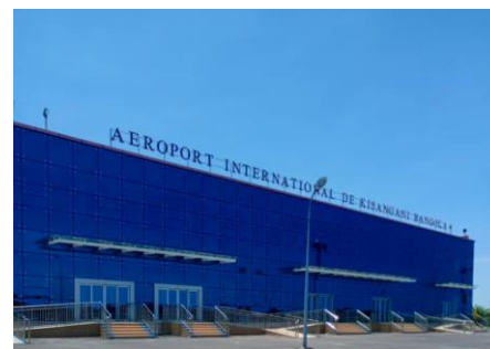
New Kisangani Terminal
