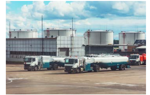
Airport Fuel Farm
