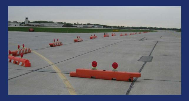
Unserviceablity markers shall be placed at intervals sufficiently close so as to delineate the unserviceable area.
