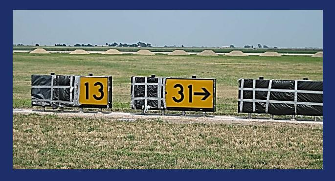
Signs for closed areas should be covered or removed so as not to provide misleading or confusing information to pilots, especially at night.
