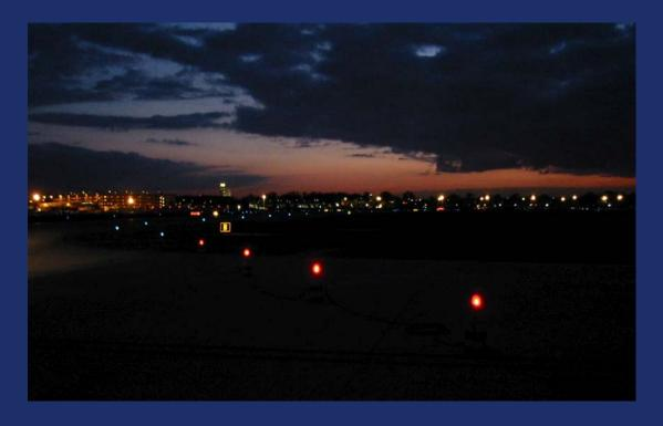
During aerodrome inspections, Inspectors should conduct night inspections of construction areas to ensure that unserviceability markers and lights are adequate and operable to keep aircraft out of construction areas.
