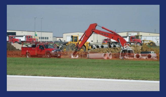
Installing a construction fence along the boundary of the protected portion of the runway safety area is an effective method of identifying construction limits and preventing inadvertent access into the runway strip.
