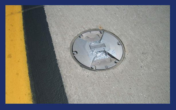
If taxiway center line lights lead into a closed area, the light fixtures should be covered if the lights cannot be disconnected or turned off.
