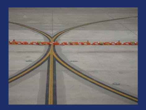
Construction vehicles normally drive through barricades to enter and leave construction sites. Installing barricades close together is an effective measure for preventing vehicles from inadvertently entering an active portion of the movement area.
