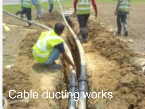
Airfield lighting cabling and pit servicing
