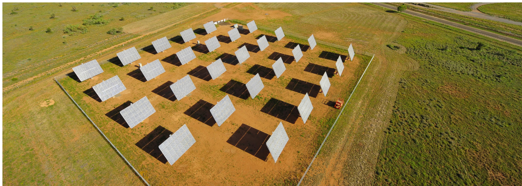
Solar tracking arrays at Alice Springs Airport
