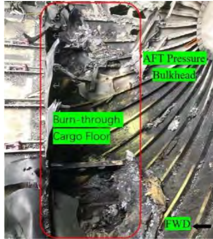
Figure 9 Burn-through Cargo Floor
