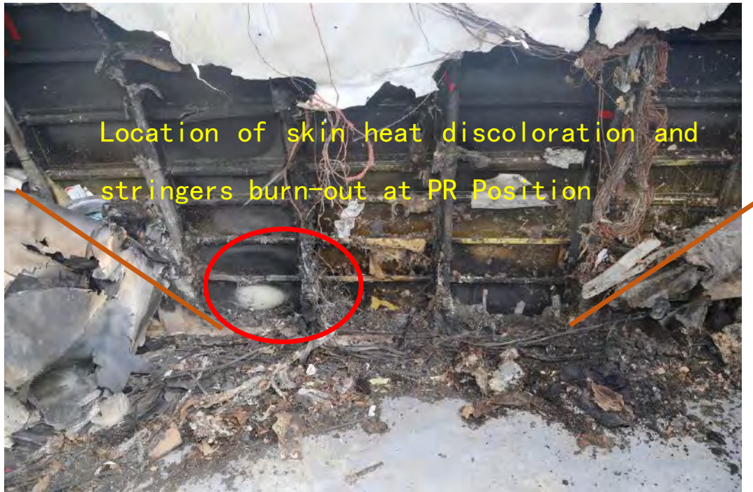
Figure 67 Details of Fire Damage at PR Position (Interior View)
