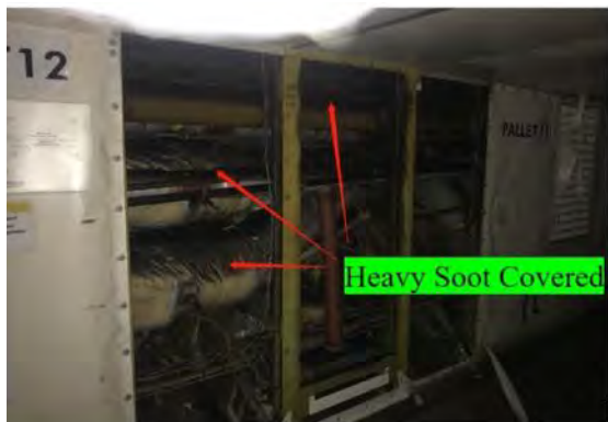
Figure 11 Inside the Lower Hold Side Wall
